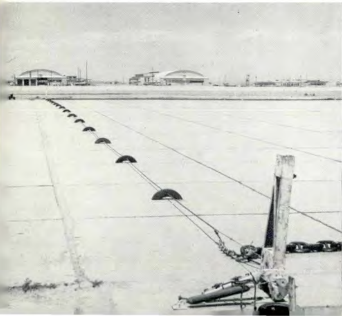
Above. The F-84 installation shows a hydraulically operated hook. Below. If arrestor cable is installed permanently above ground, tire casing supports can be used to keep cable 3 1/2-6 inches off runway.
